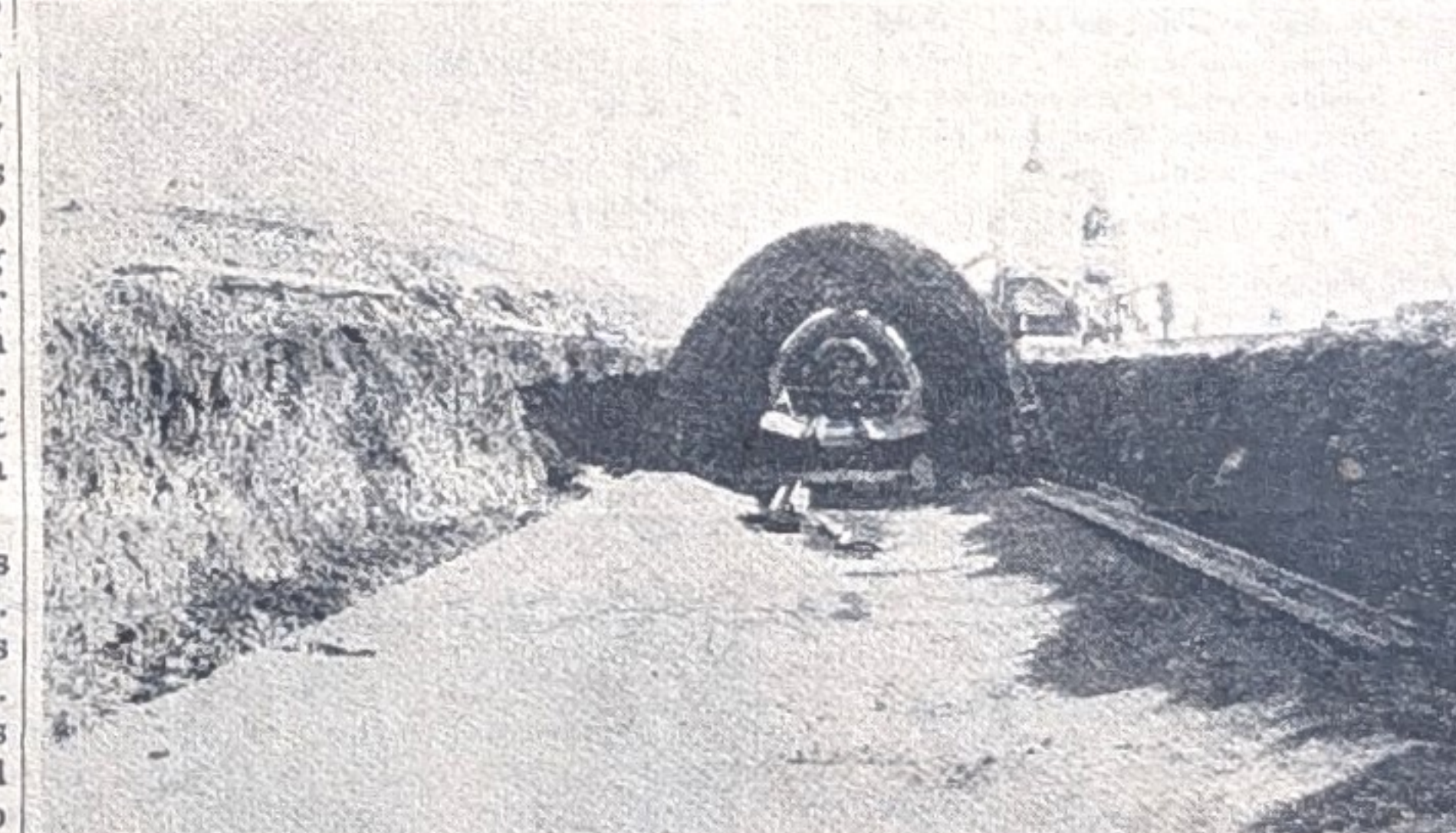
FRONT VIEW OF AQUEDUCT: here is a front view of the huge pipe. It is over six feet high, built of re-enforced concrete. Where the drop was sufficient smaller round pipe was used. Each section is joined to the next by a copper u-shaped joiner that allows the pipe to contract and expand a bit. The track in the pipe is to move the inside part of the form. Forms were very heavy, were built of steel. Only 3 sets of forms were used in the construction of the entire 97 miles.
